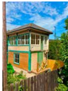
Renovation work is underway at Uckfield's old signal box to create a micropub but red tape is causing delays
